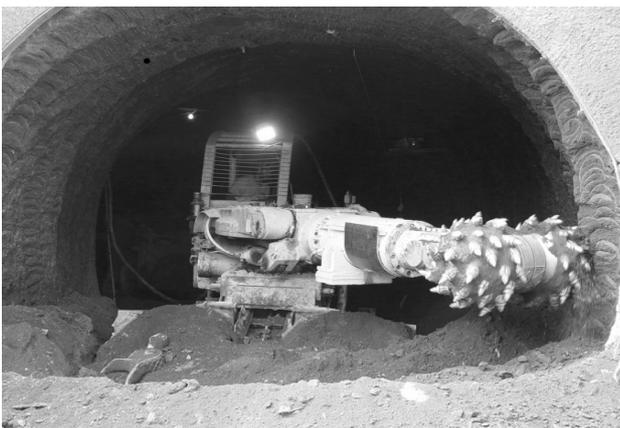
Fig. 3. A roadheader during work procedure
