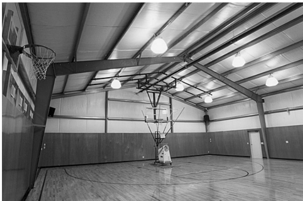
Fig. 1. An interior of a one-storeyed building
