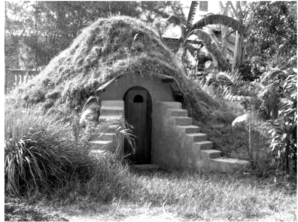
Pic. 5. Example of earth-bag construction
