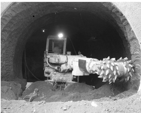
Pic. 3. A roadheader during work procedure
