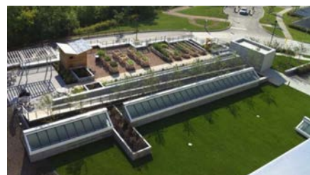
Рис. 6. UVM Medical Center Radiation Oncology Building , Vermont
