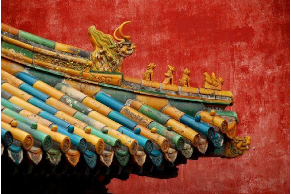
Fig.2. The fragment of the roof of the secondary pavilion with ceramic tiles and animal figures. The number of figures indicates the status of the building. (From the funds of Chang Peng).
