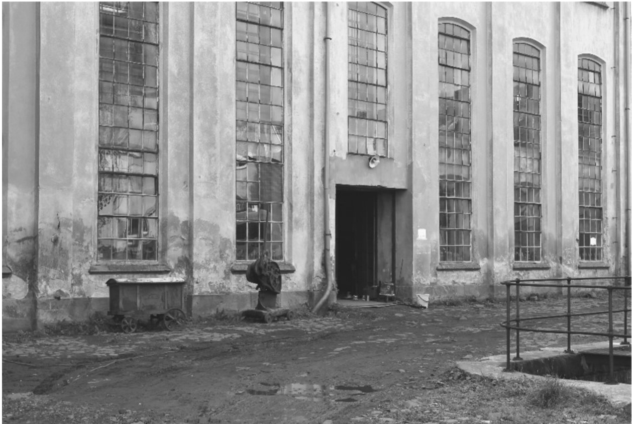
Fig. 2. Facade of the first mechanical weaving factory in Bohemia called "Továrna Mastných", Lomnice nad Popelkou (author's photo)
