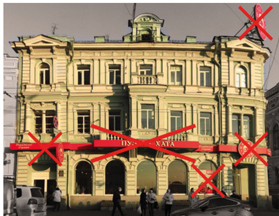
a) Incorrect advertising signs
